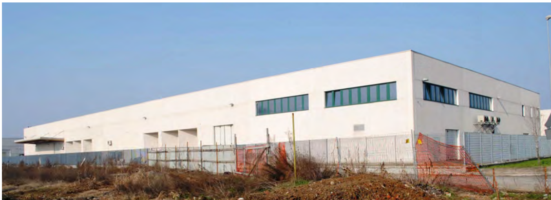
Industrial shed – Vellezzo Bellini (PV)
